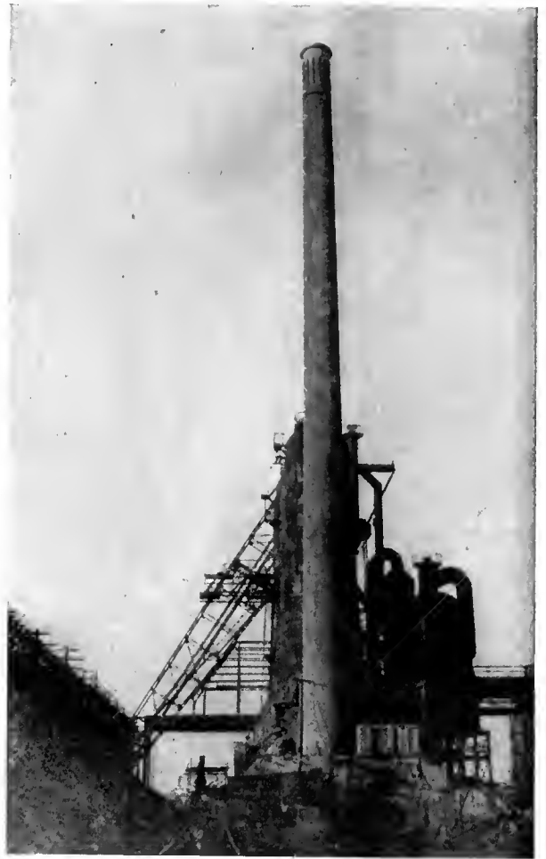
BLAST FURNACE CHIMNEY
